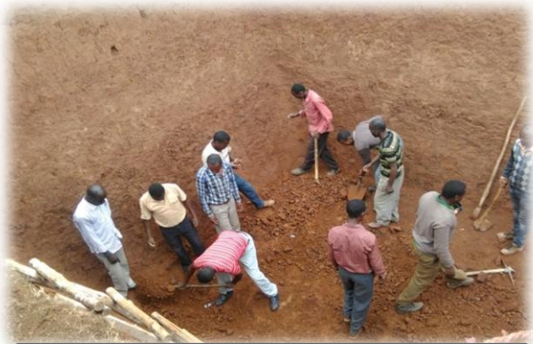
Community participation during the construction
